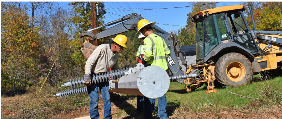
Contractors attach insulators to a new pole before they erect it as they work on a transmission line upgrade this year.
