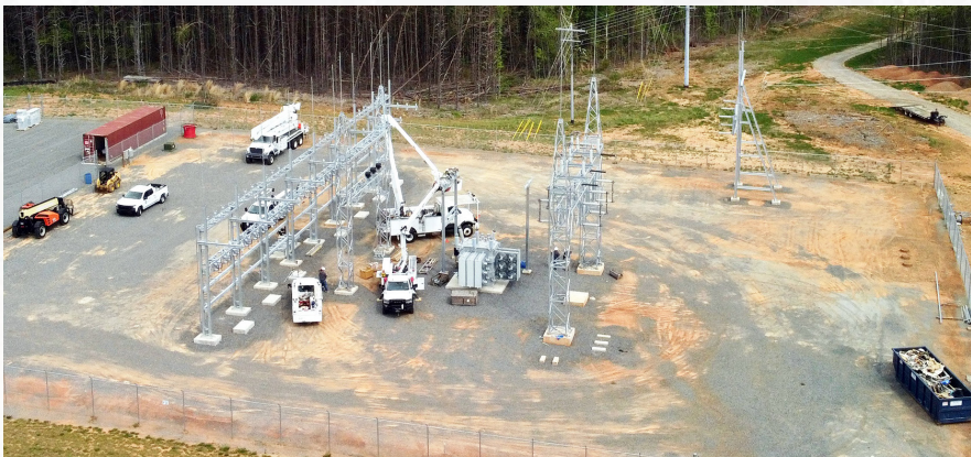
This aerial shot from a drone shows work continuing on the Double Creek substation being built on N.C. 268 northeast of Pilot Mountain in Stokes County. The project will help ease the load and burden on substations in the Westfield, Francisco and Hanging Rock areas, as well as provide a way to back feed distribution circuits to help reduce outage times and the number of members affected and to allow for additional capacity for future growth in these areas.
